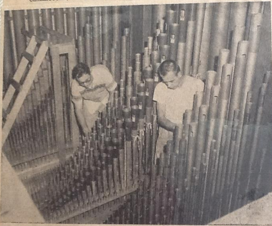
Finishing touches on the pipes for the new First Presbyterial Church organ were being made Friday by Maurice Plog (left) and Ed Notter of the Wicks Organ Co., Highland, Ill. More than 2,000 pipes, ranging in length from one-half inch to more than 20 feet, were placed in two soundproof chambers at the rear of the chancel. (Gazette Photo by Robert D. West).
